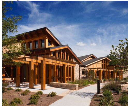
Figura 19 – WILSON HOSPICE HOUSE
