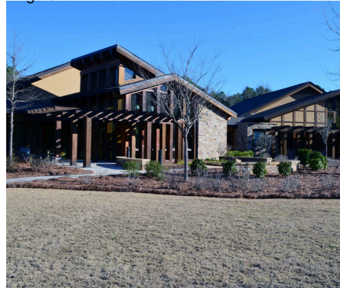
Figura 23 – WILSON HOSPICE HOUSE
