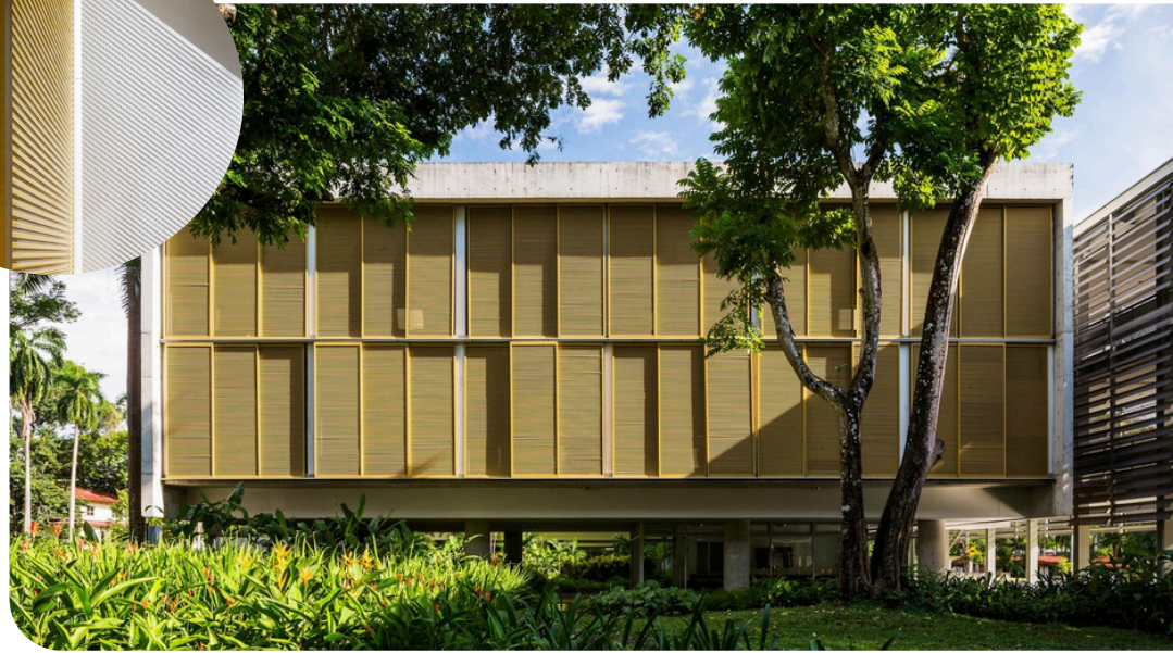
Figura 16- Fachada principal com brises
