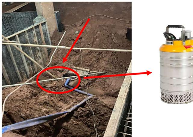
**Figura 2: Bomba submersa ASI 500**
