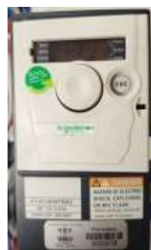
Fig. 4. Inversor altivar 312 (ATV 312)
