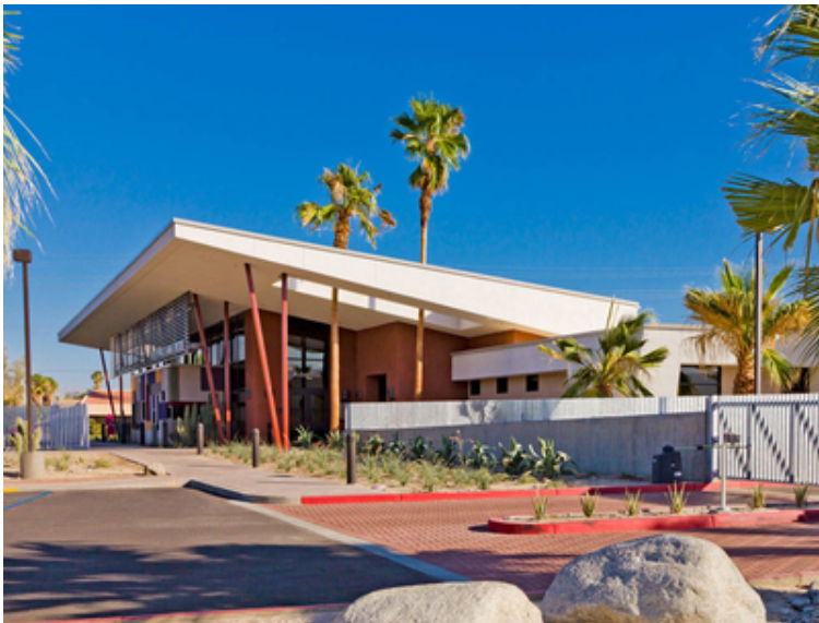
Figura 57: Palm Springs Animal Care Facility. Fonte: Archdaily.
