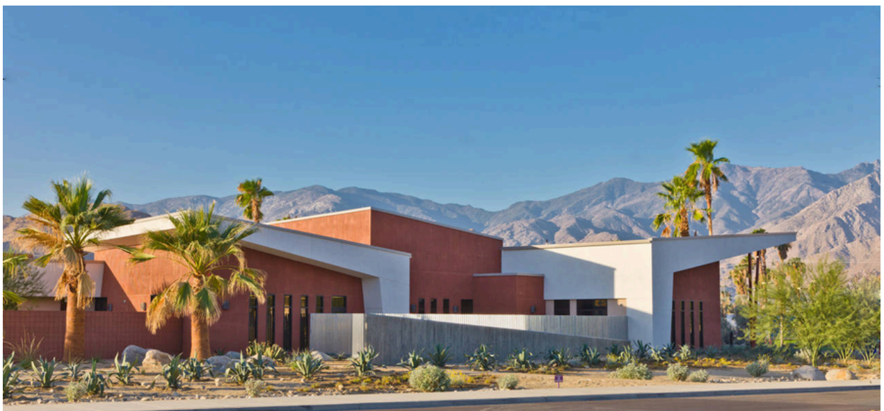
Figura 59: Palm Springs Animal Care Facility. Fonte: Archdaily.
