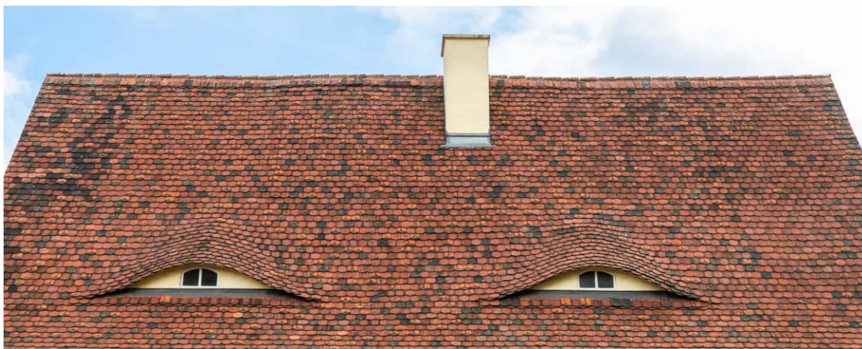
Ilustração 3 Telhado estilo fachwerk com janela-sótão em forma de olho Fonte: ADOBE STOCK (2021). Disponível em: https://stock.adobe.com/pt/images/old-beautiful-european-german-fachwerk-building-rooftop-with-eye-shaped-windows-and-chimney-typical-traditional-ancient-house-roof-architecture-in-europe-funny-face-shaped-pareidolia-facade/525107304 . Acesso em: 28/11/2025
